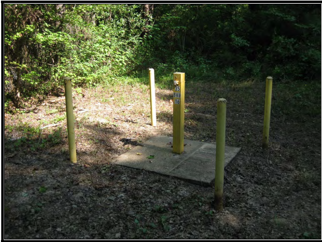
PHOTO 13: 35BWW16 DATE: August 7, 2019
