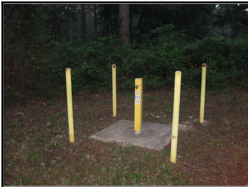
PHOTO 16: 35BWW19 DATE: August 5, 2019
