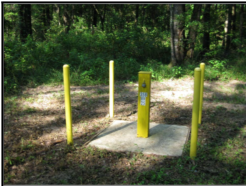
PHOTO 20: 35BWW25 DATE: August 7, 2019
