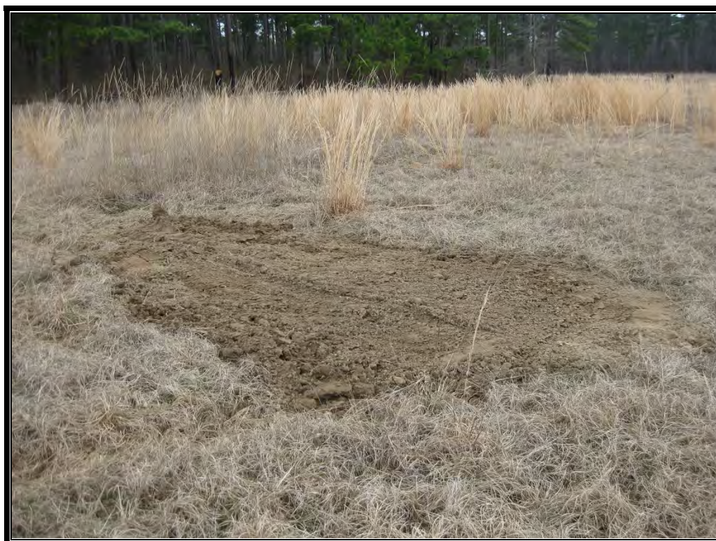
PHOTO 12: Repair of Holes in Cover DATE: February 1, 2019
