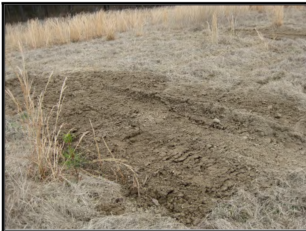
PHOTO 11: Repair of Holes in Cover DATE: February 1, 2019
