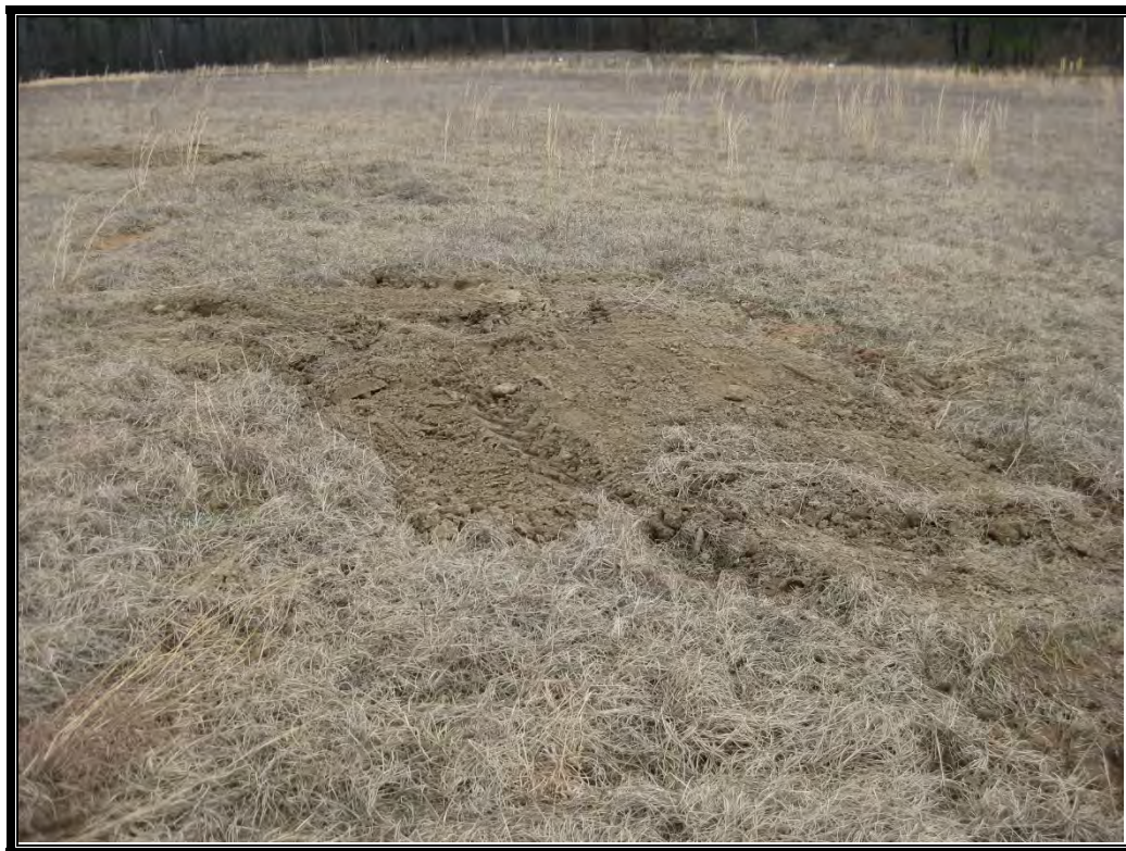
PHOTO 13: Repair of Holes in Landfill Cover DATE: February 1, 2019
