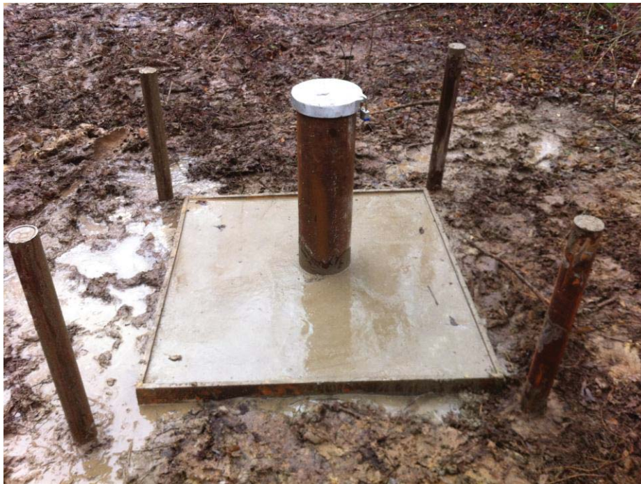
Surface Completion of MW 35BWW11
