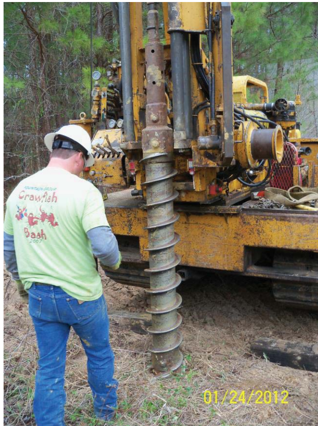
Installation of MW 35BWW11
