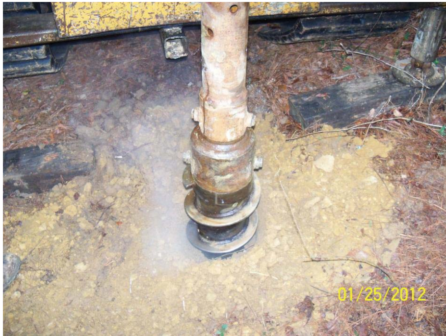
Installation of MW 35BWW09
