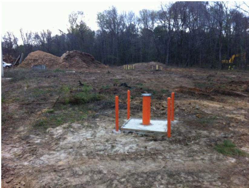
Completed MW 35BWW11
