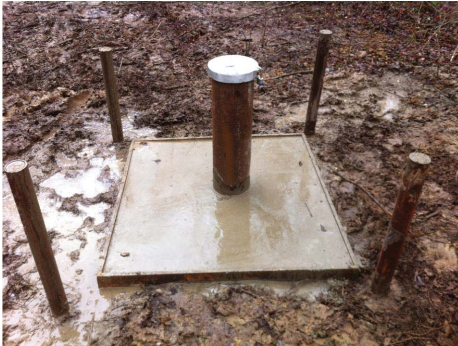
Surface Completion of MW 35BWW11
