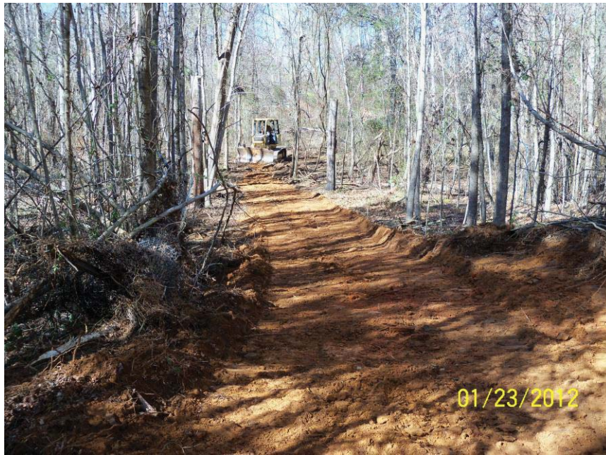
Clearing for MW 35BWW14
